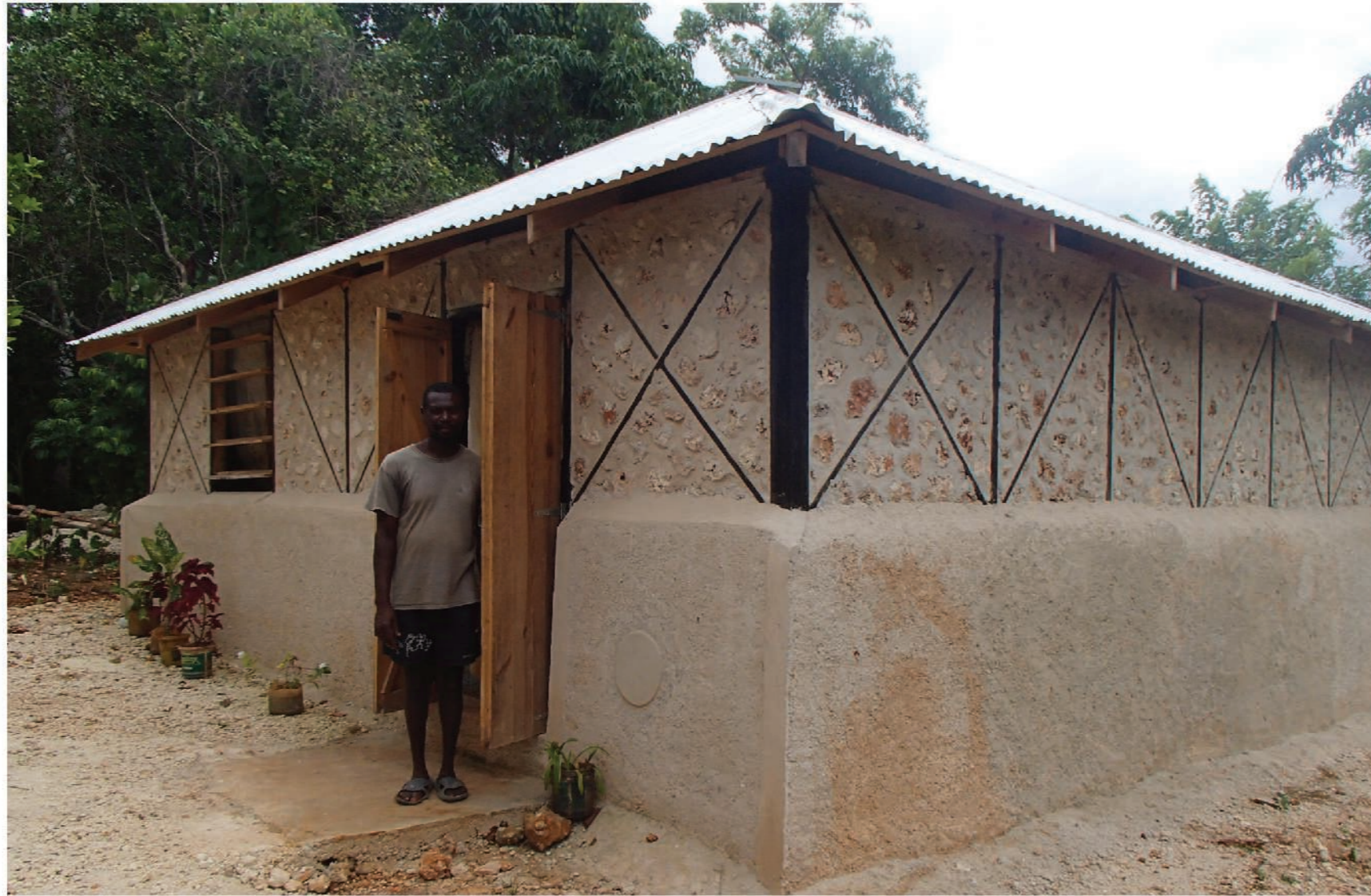
RECONSTRUCTION OF A SUSTAINABLE HABITAT USING CONFINED STONE WALL TECHNOLOGY
